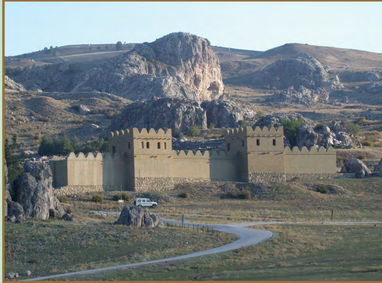
Figure 3. The 65 m long reconstruction of the mud brick city wall of Hattuša.
