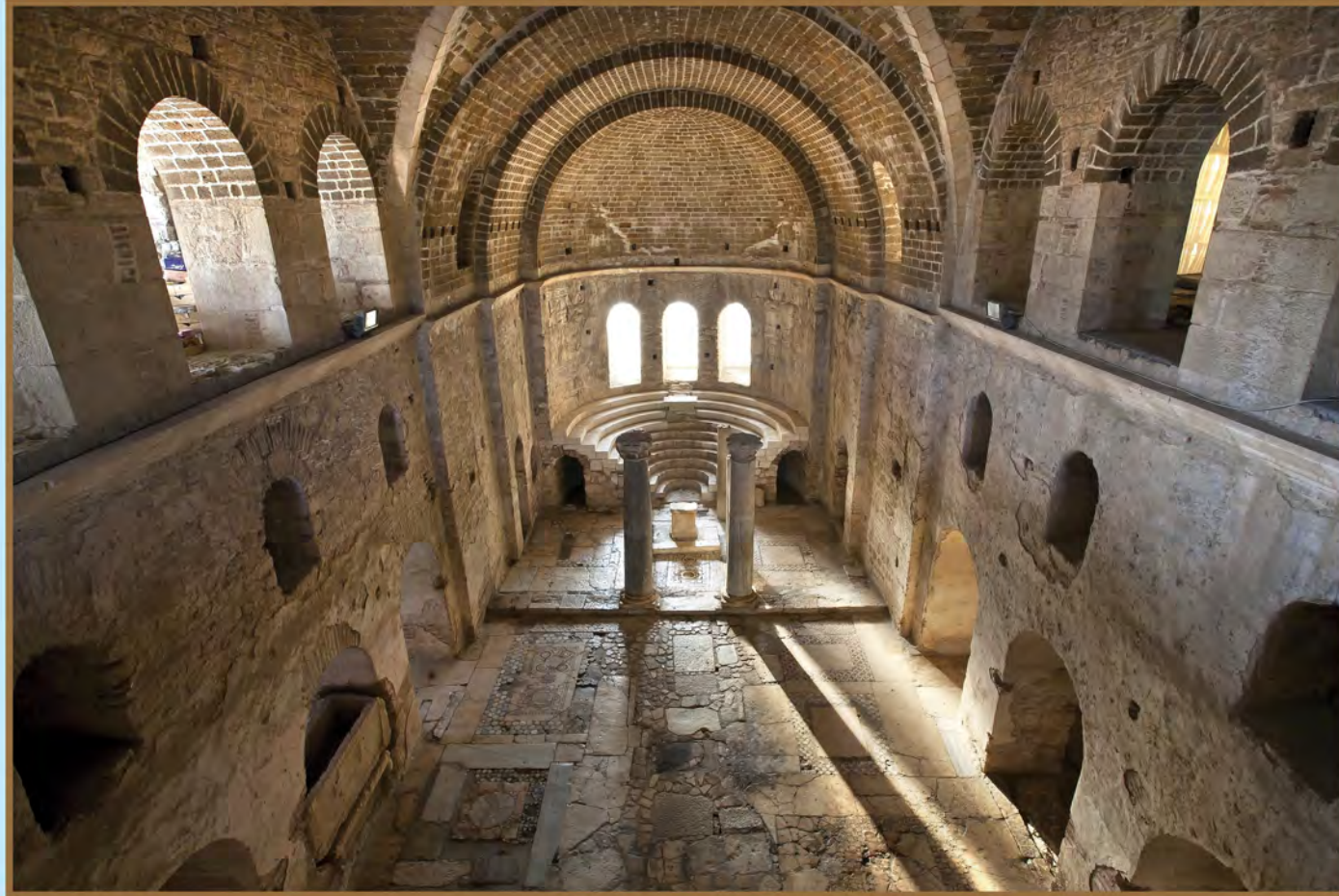
Figure 7. Church of St. Nicholas in Demre, Naos, looking east
